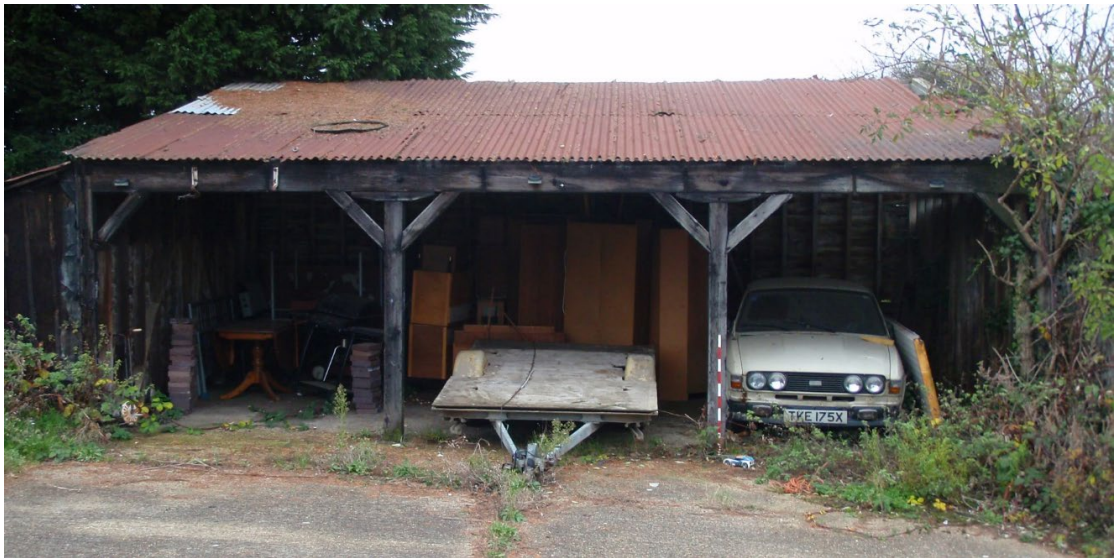
Plate 17: View of cart shed (looking north west)
