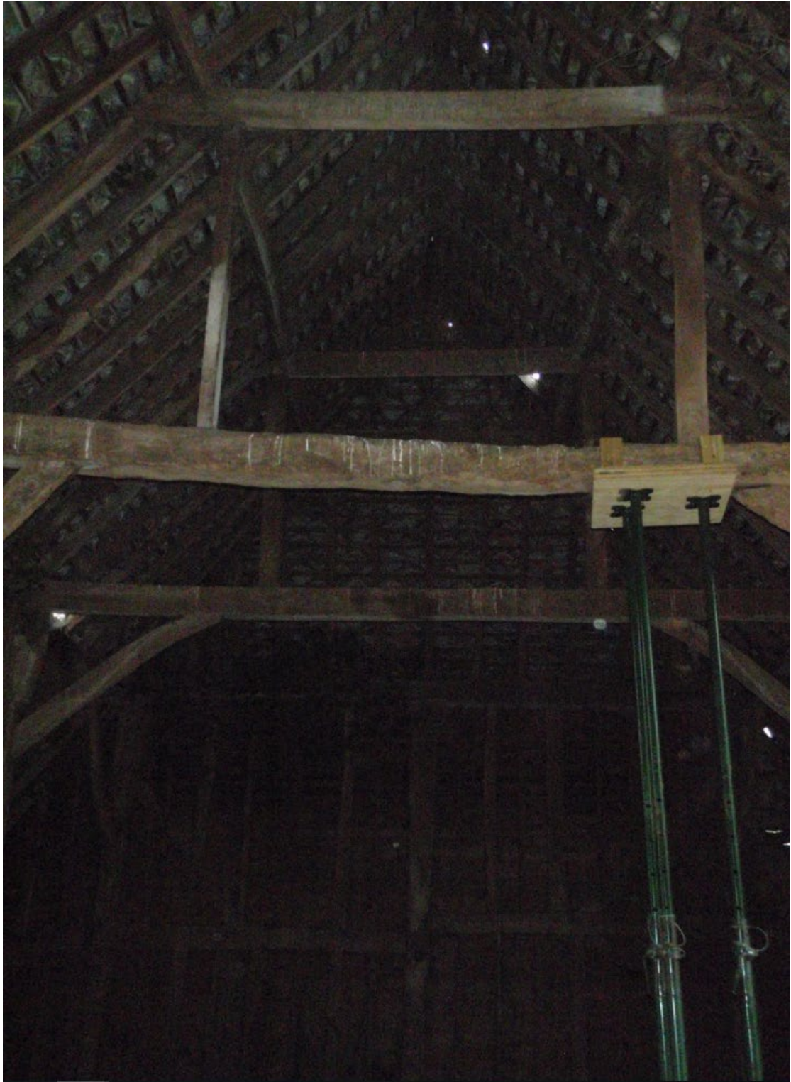
Plate 15: Interior view of the south western half of the barn
