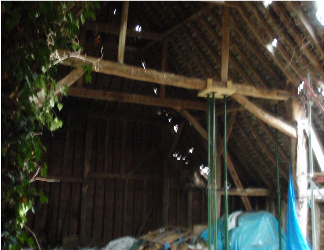
Plate 13: Interior of barn (looking south west)
