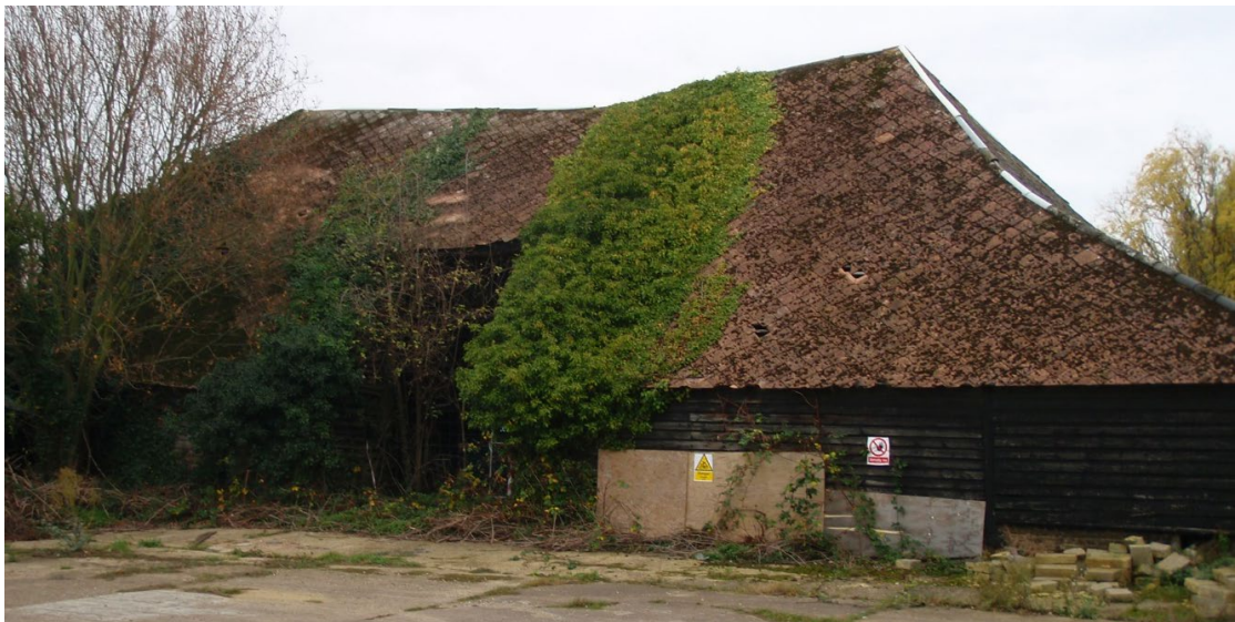
Plate 10: Barn (looking east)
