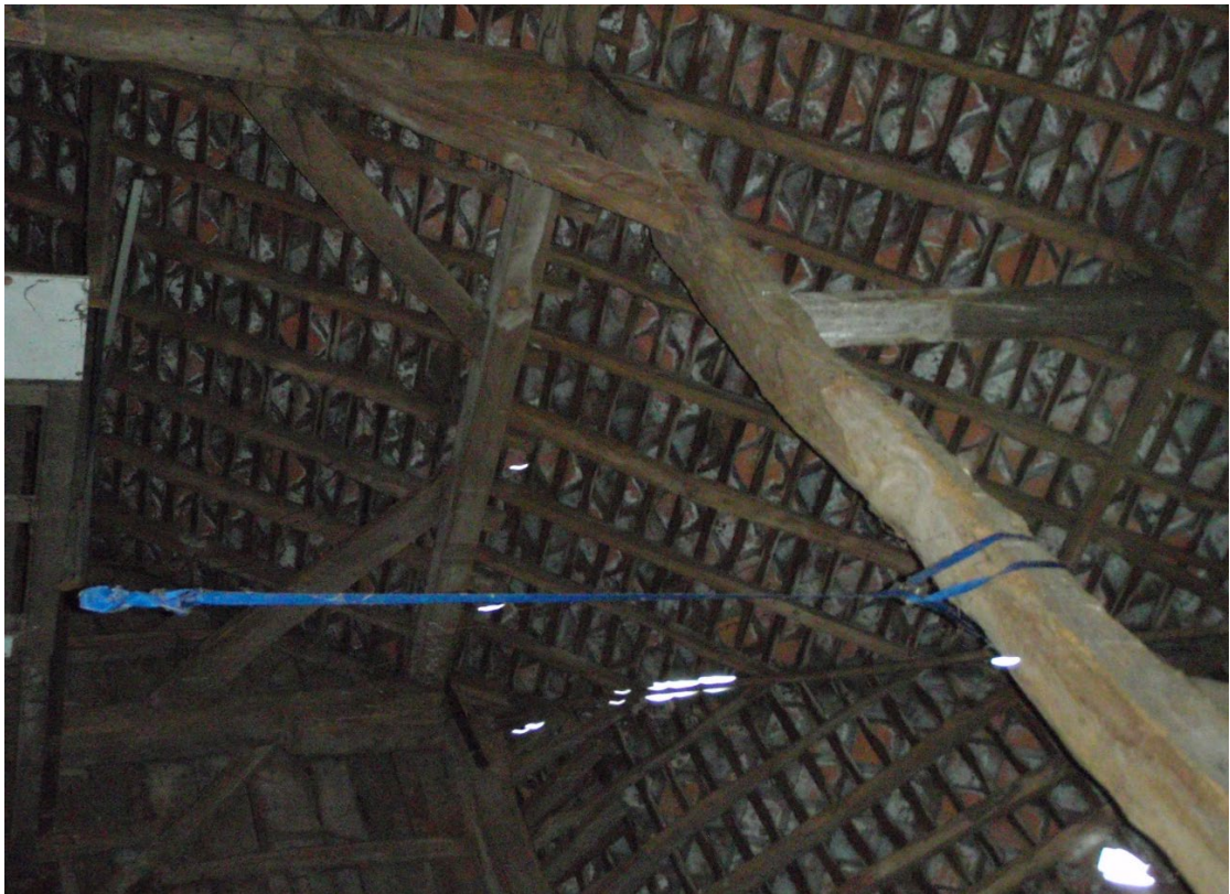
Plate 14: Close up of one of the trusses of the interior of the barn
